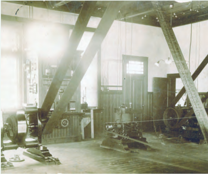
These two rare photos show the interior of the electrical plant at Bedloe's Island, circa 1890. The early Wood Dynamo Electric Machine used to generate the electricity to light the Statue and island's buildings is seen at the far left of the photos. Charles wrote of getting burned by flying sparks if he got too close. (Courtesy Lehman College, CUNY. Charles Miller Collection.)
