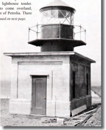
This photo was taken in 1912 immediately after the Punta Gorda Lighthouse tower was completed and before the lens was installed in the lantern. (Photo courtesy U.S. Coast Guard.)
