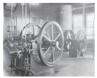
The interior of the fog signal building at Punta Gorda Lighthouse showing the engines and air compressors as they appeared in 1916. (Photo courtesy of the U.S. Lighthouse Society.)
